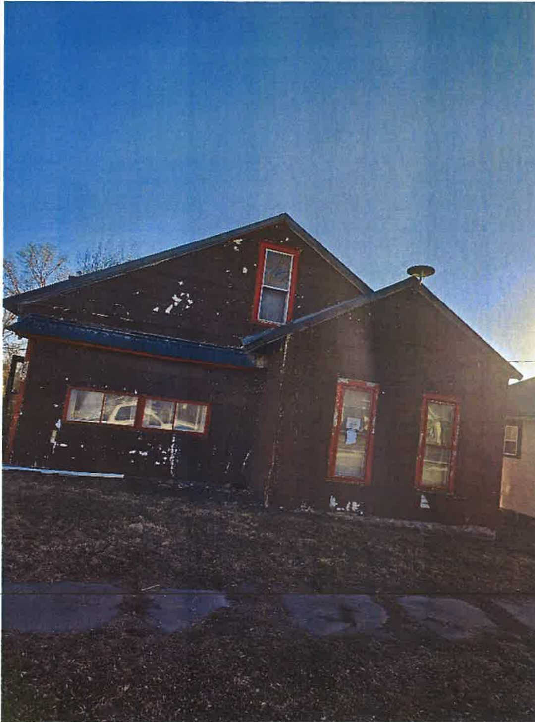
1550 Mable Ottumwa, Iowa Asbestos Removal, Demolition and Disposal Bid Packet
