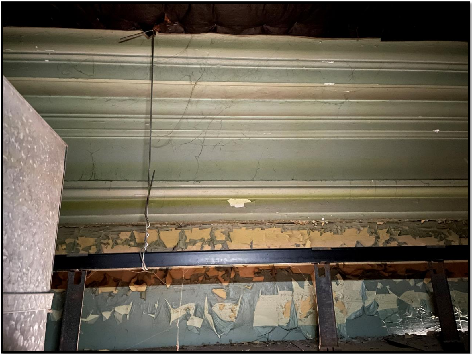
Original Ceiling Details Above Drop Ceiling (Typical)
