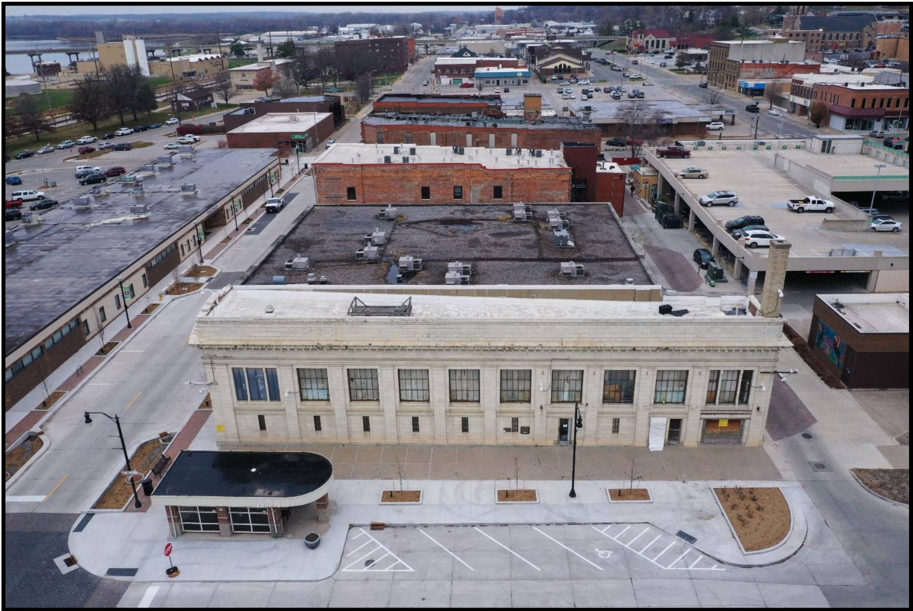
Side & Roof (Current)
