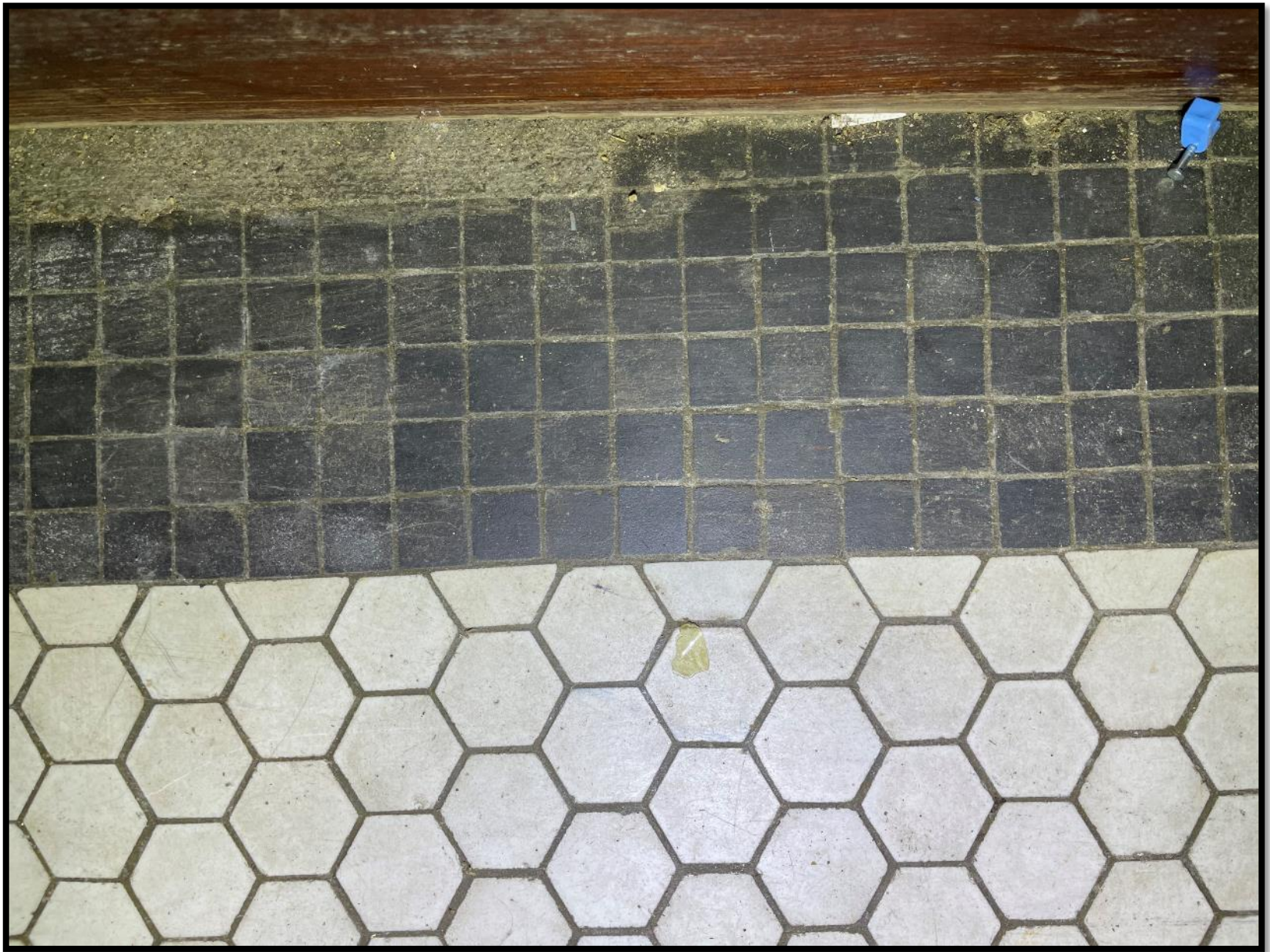
Exposed First Floor Tile (Typical)
