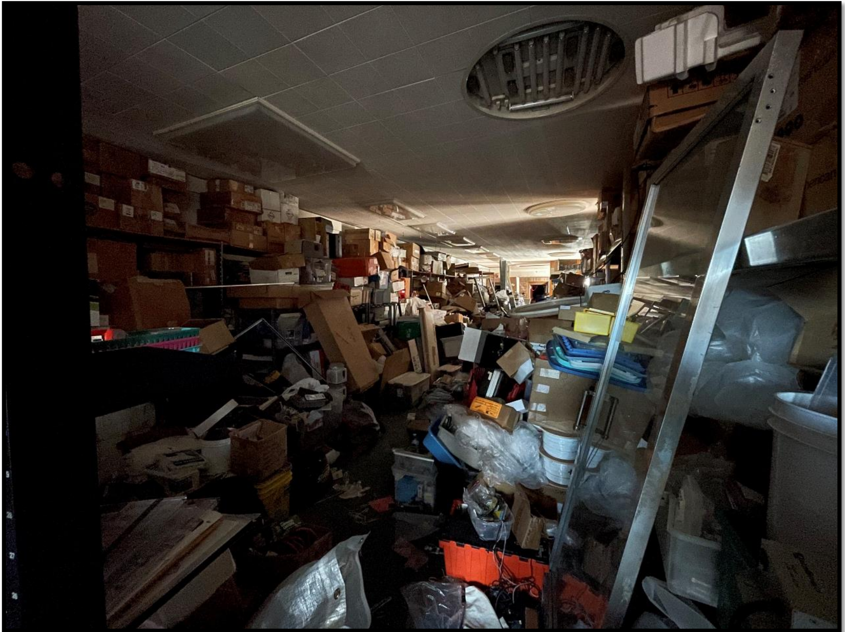
First Floor "Lobby" View – Looking to Rear (Before Cleaning)
