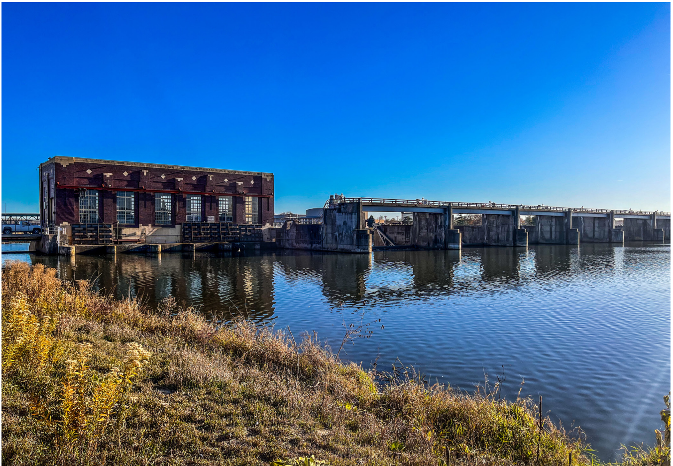
Ottumwa Historic Hydro-Electric Plant, 1930-1931.
